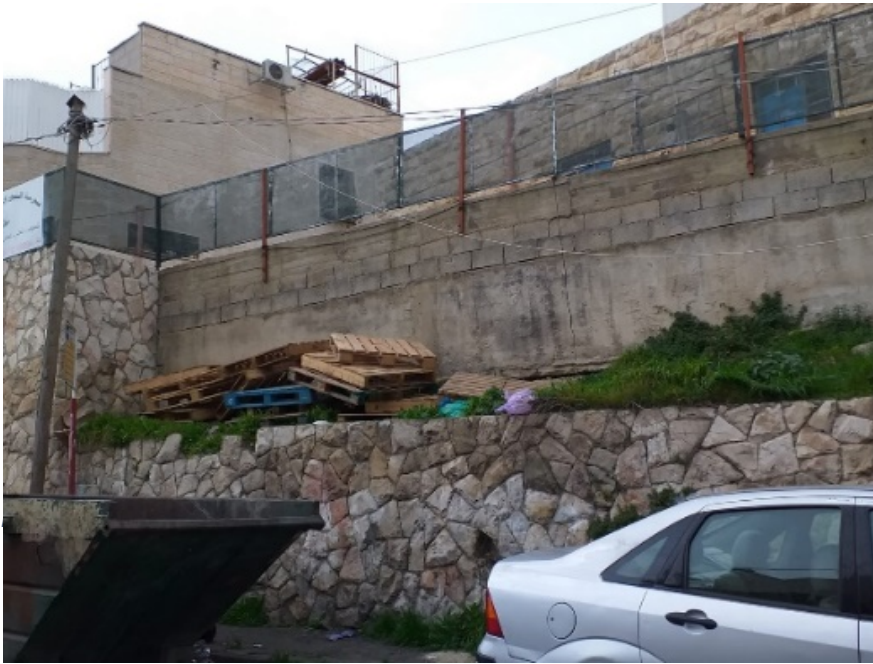
Figure 3: Exposed electricity lines in A-Thuri
